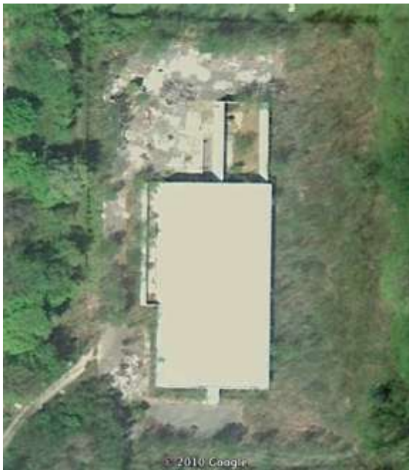
2010 Google Earth Aerial
