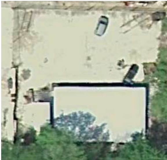
2010 Google Earth Aerial
