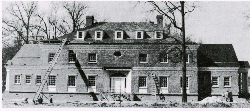
94. Pi Kappa Alpha, national headquarters by George Mahoney, under construction, 1945.
