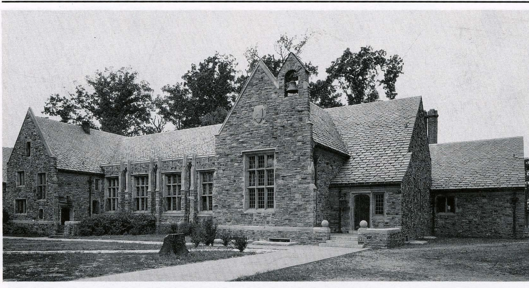
29. Neely Hall and Refectory, 1925.
