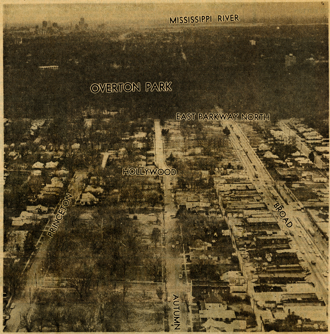
Buildings Between Autumn And Princeton Have Been Removed For Expressway Approach To Park
