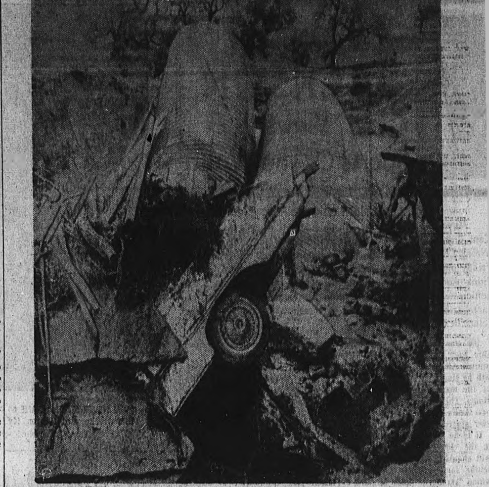
A COLLAPSED ROADWAY and a half-buried auto give you an idea of the havoc caused by Southern California's heaviest rains in three decades. This scene is at Thousand Oaks.
