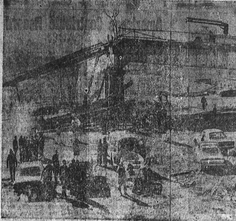
RESCUE OPERATIONS at Point Pleasant, W. Va., landside part of the bridge still upright. The after collapse of the Ohio River bridge show bridge crumpled into the river with a rush-hour load of traffic.
