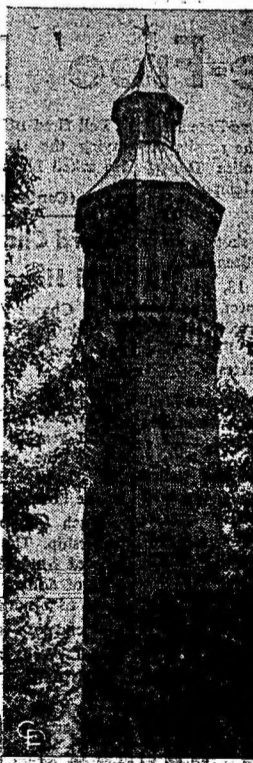
The High Bridge Tower Today. designed to protect its interior tank from forming ice in winter, were cleaned and joints re-pointed.
