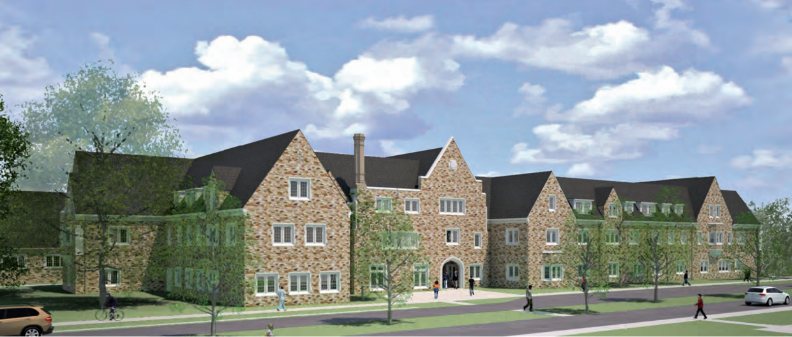
Rhodes' newest residence halls facing Bailey Lane
