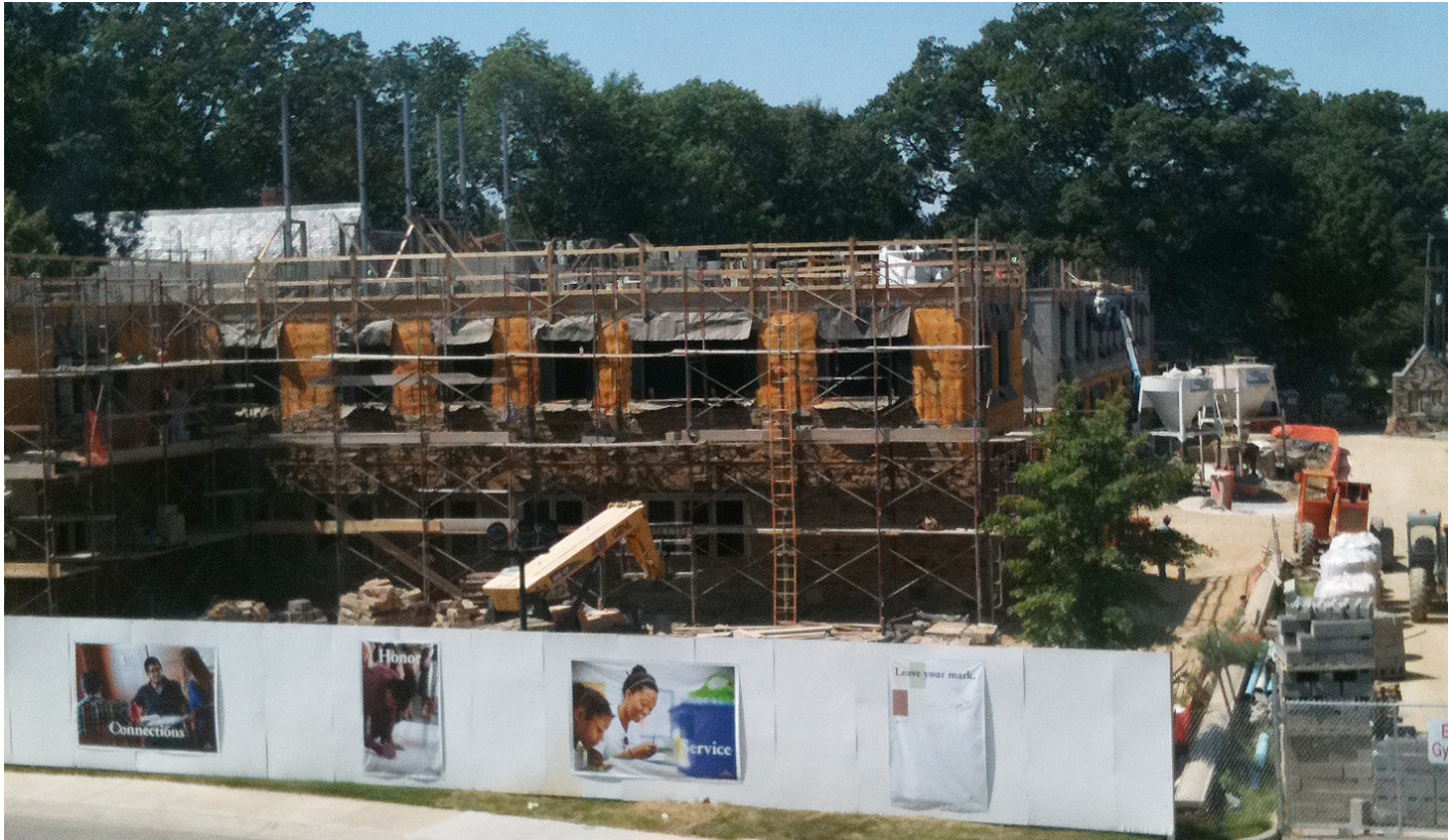
Construction photo courtesy of Swati Pandita
