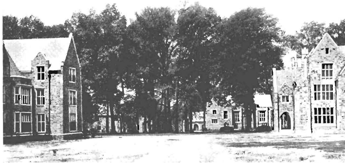
A Partial View of Campus and Buildings.
