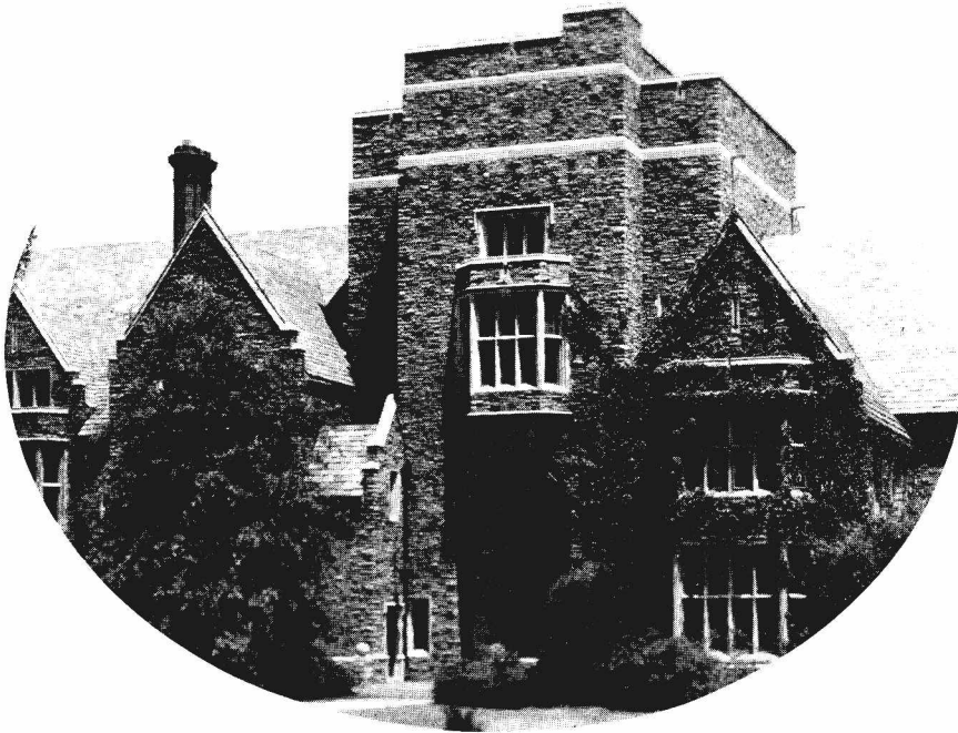
Palmer Hall Main Entrance
