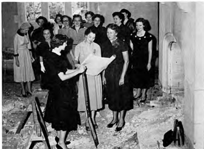
Vi dug up the floor all by herself!
