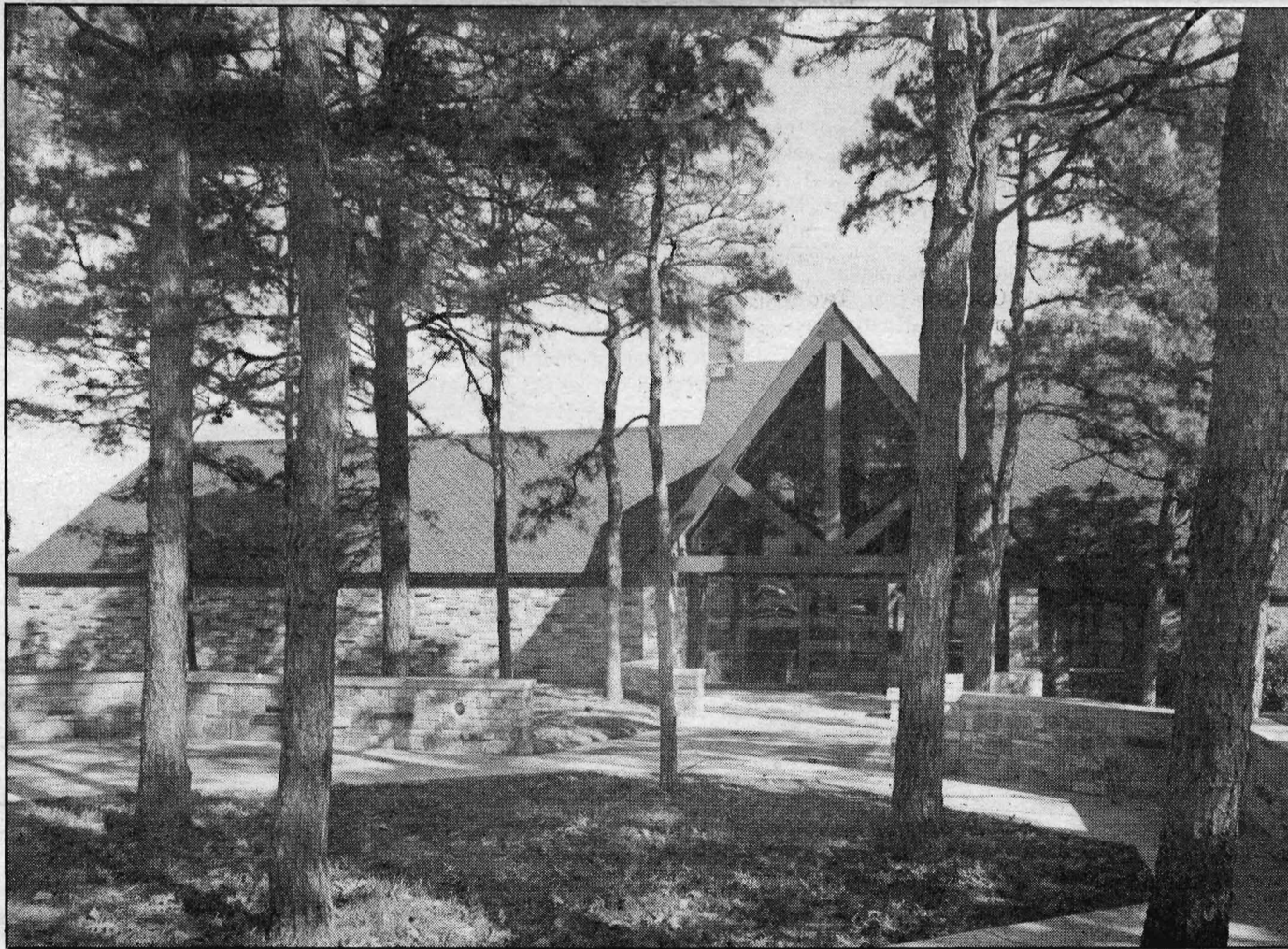
PLAYHOUSE IN THE PINES — The new McCoy Theatre, designed by Met Crump of Taylor and Crump Architects rises gracefully in a grove of pines on the northeast side of campus. "The two story entrance with its heavy wood roofed truss is intended to provide an element of strength and boldness of character" says architect Crump. The glass-fronted entrance is approached through a semi-enclosed courtyard. The actual theatre stretches to the left. (photo by Alan Karchmer).
