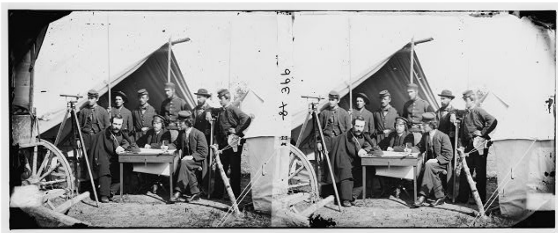
15 2 Detail of Yorktown, Va., vicinity. Topographical engineers, Camp Winfield Scott Taken from: http://memory.loc.gov/service/pnp/cwpb/00100/00124v.jpg
