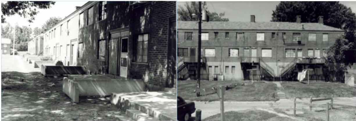
Image 4. LeMoyne Gardens before demolition. Source: The City of Memphis Housing Community and Development Department.
