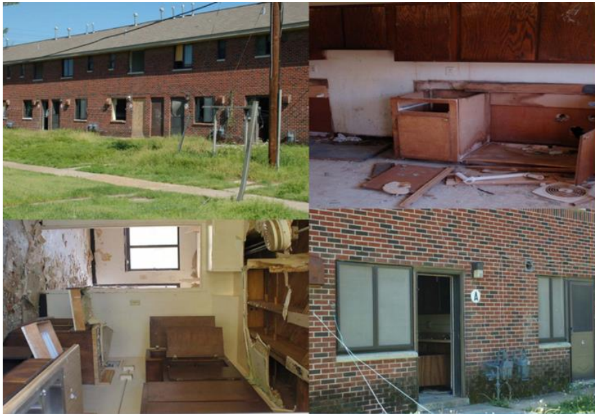
Image 2. Cleaborn Homes before demolition.
