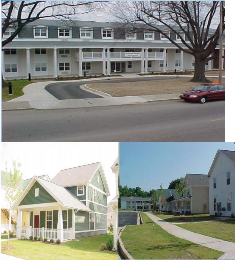
Image 5. College Park after the redevelopment. Source: The City of Memphis Housing Community and Development Department
