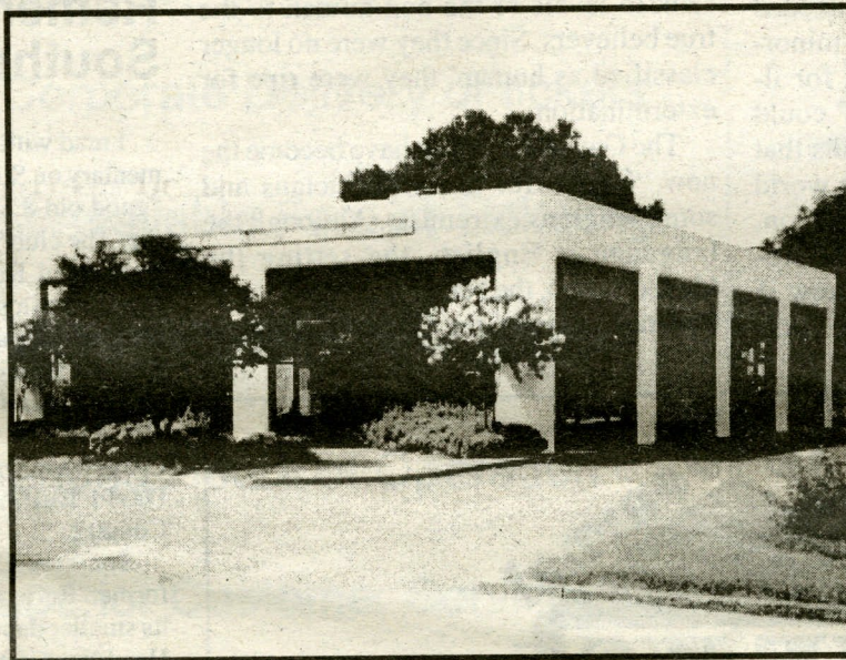
Holy Trinity Community Church has purchased this 5000 square foot building at 3430 Summer Ave. The building was built in 1963. Initial plans include renovating the existing space for church use; long-term plans call for a sanctuary addition to the building.
