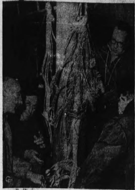
OUT OF ORDER—New Jersey Bell Telephone Company supervisors repair a cable near Newark Airport, one of 28 found slashed over the state after Communications Workers struck.
