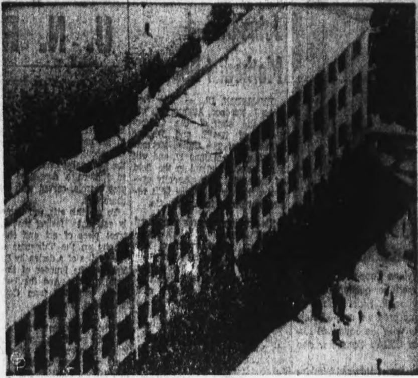
THE WORLD'S MOST POWERFUL EARTHQUAKE since the Alaska shock of 1964 left this Hakodate University building in Japan broken like a child's toy. Hakodate is a large city on Kakkado, Japan's northernmost main island. The quake destroyed some 1,200 homes and left more than 40 persons dead.
