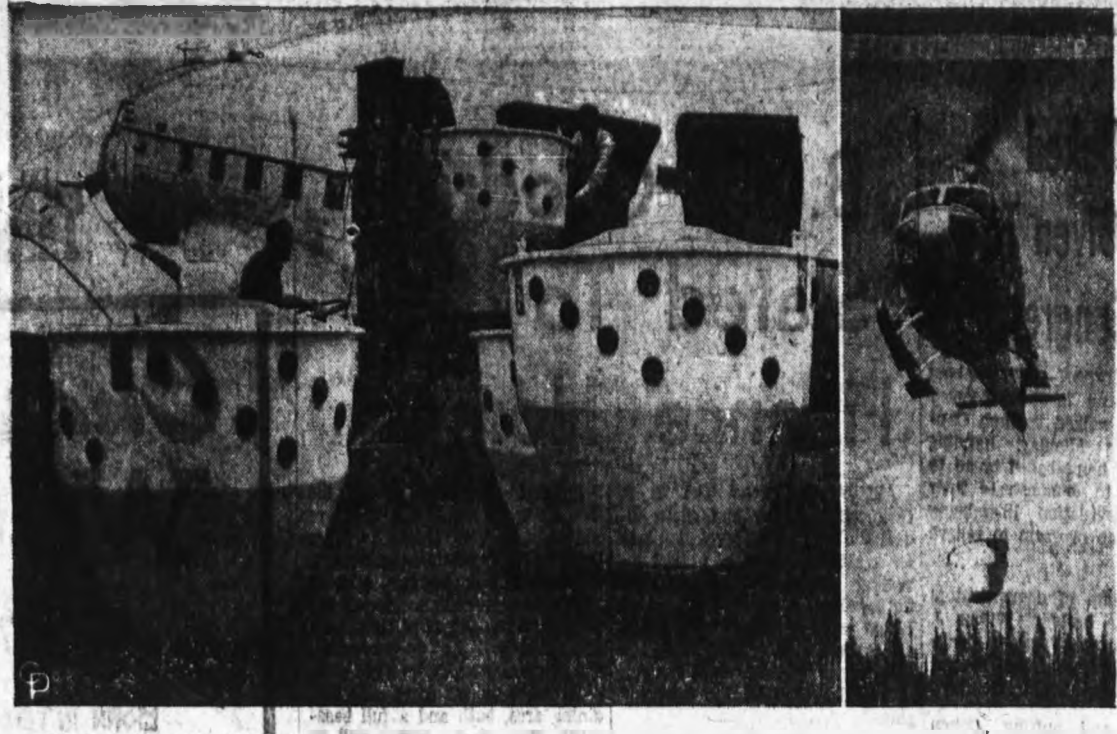
DOUSING THE ROCKET'S RED GLAZE - Fiberglass 'buckets' the U. S. Forest Service uses to fight fires (right) by helicopter are being airtight (left) to Vietnam for use against fires started by rocket and mortar attacks.
