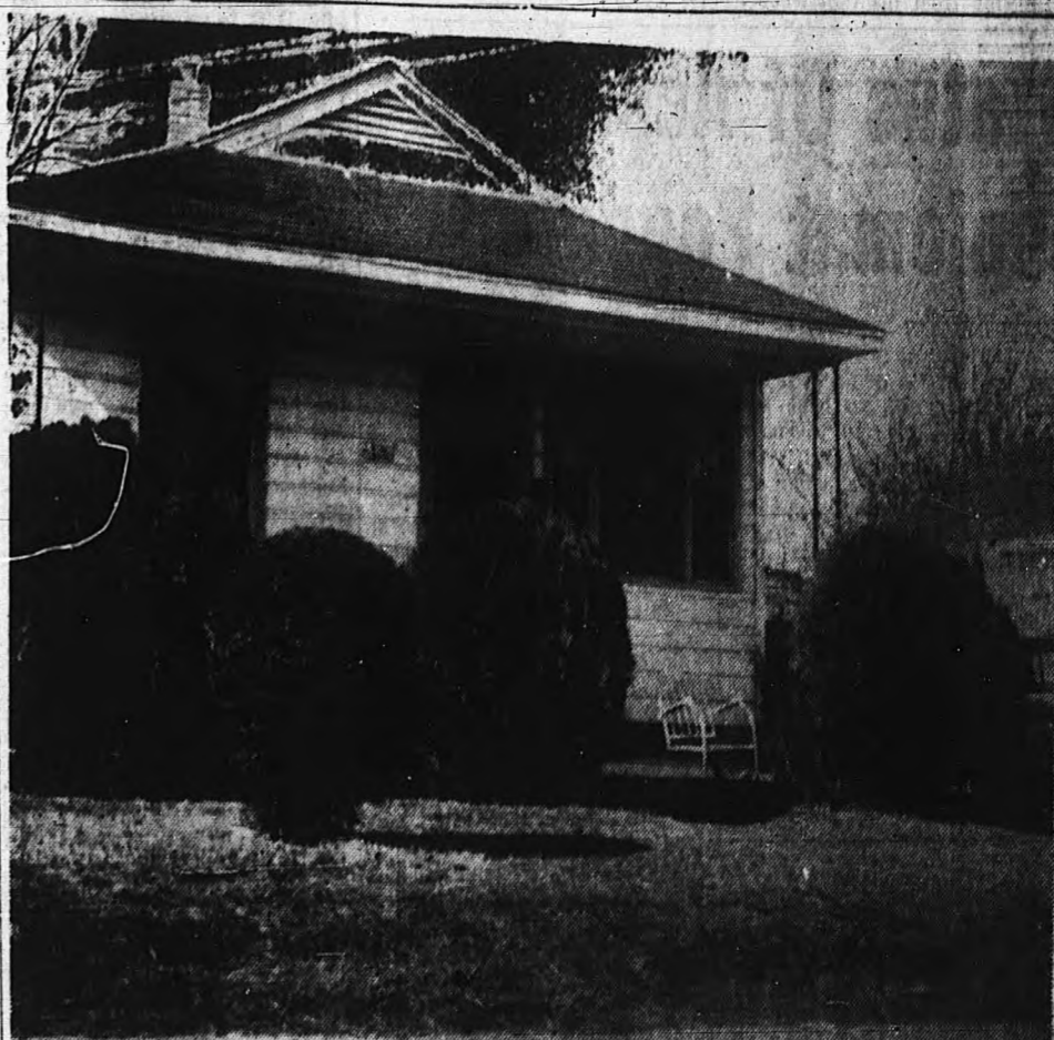
THE LONELY PORTER HOME —There is a ghostly quietness in and around this neat-looking house at 1701 Ash Street this week. It was the home of Mr. and Mrs. Eli Porter, Sr., and their five sons, ages 3 to 12. The father and the five boys were buried Sunday, all victims of fumes from an unvented gas stove. Mrs. Porter, also felled by the fumes, is the only surviving member of the family.
