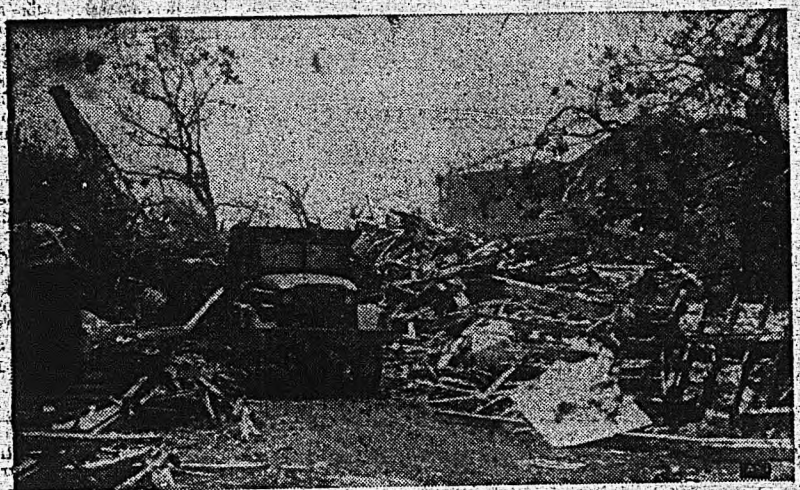
DEBRIS IS LOADED on trucks by heavy equipment operated by Army National Guardsmen during the aftermath following hurricane Camille. National Guardsmen participated in rescue, security and cleanup operations. In addition, they provided transportation, communication and electric power. The Mississippi National Guard established a refugee center at Camp Shelby, Miss., a facility capable of accommodating 4,000 persons.
