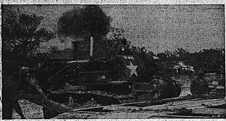
CLEARING A HIGHWAY. A medium tractor, D-7, operated by soldiers of the 818th Engineer Battalion (Combat) clears debris from a town in the Gulfport area, Miss. The rapid opening of roads speeded the evacuation of casualties from the disaster sites.
