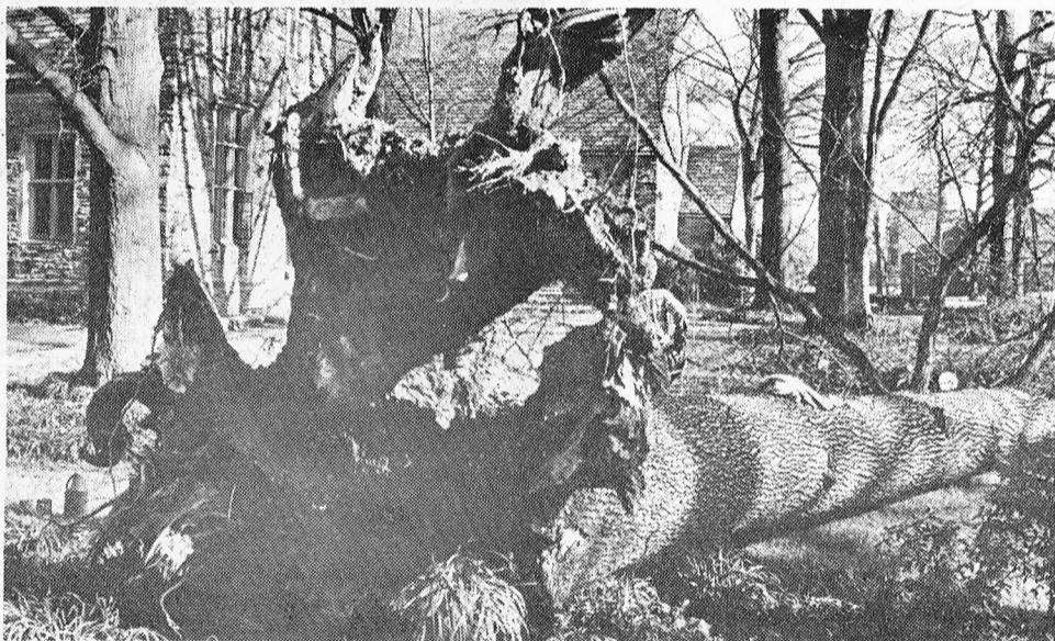
The storm that struck last April 7 left trees uprooted and damages in excess of $20,000 to the campus. Most of the damage was to the roof of Bellingrath and the greenhouse atop the Math Building. Photo by John Peeples.
