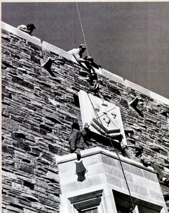
Installing the college seal on the Peyton Nalle Rhodes Physics Tower in 1968
