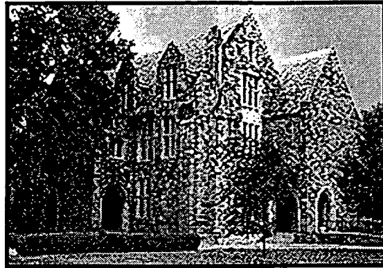
Berthold S. Kennedy Hall Dedicated October 19, 1968
