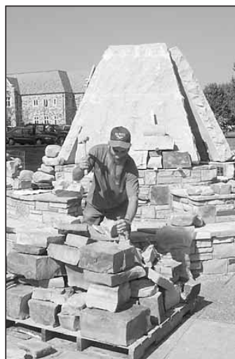
Bobby Parnell of W.A. Fortner Masonry chisels a block of Arkansas sandstone before placing it on the fountain in Garner Court.
