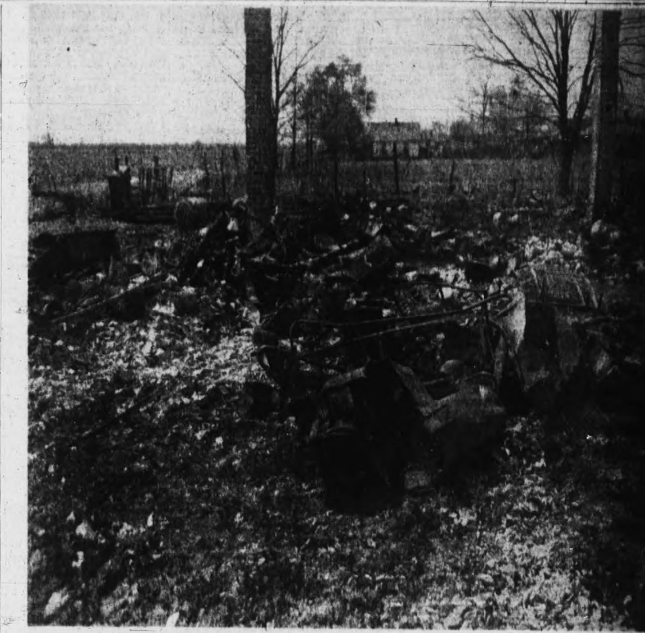
HOME DESTROYED BY FIRE —The above picture shows all that remained of the once spacious home and office of Dr. Stanley Ish, Jr., Marion Ark., physician, after fire completely destroyed the building early Sunday afternoon. Dr. and Mrs. Ish were in Hot Springs, Ark., for the week-end and learned of the tragedy when they arrived at the Little Rock
